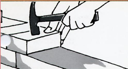
Tap the brick firmly into place with hammer against the top.
