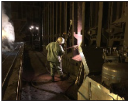
Ceramic welding from coke side bench
