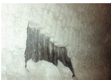
Figure two: Brick loss in a "trough" formation due to a problem with alignment.
