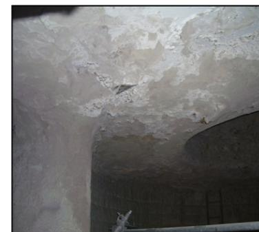
**Figure 5.** After a year of service in this bottom stage cyclone roof, QUIKTURN™ 60Z PC, which contains a zircon addition, appears in excellent condition with no cracking and good resistance to buildups.
