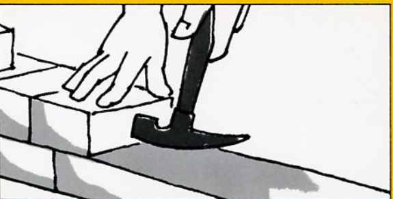
Tap brick firmly with hammer against side as shown.
